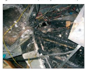
Figure 19: Fire in an air-handling unit (electrical) (courtesy of Network Rail)
