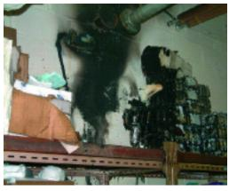
Figure 4: Fire in a storeroom (hot works) (courtesy of Network Rail)
